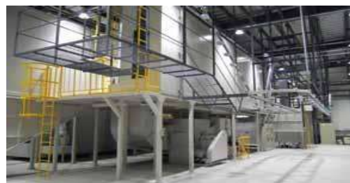
Automated coating process
